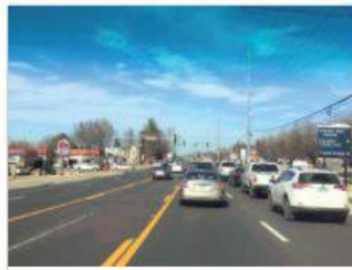
Continuous Center Turn Lane
